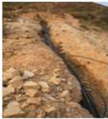
Our water project in Pipaldali is progressing well. The channels to take the pipe runs from the main collection tank to the 36 dara (standpipes) have been dug on the steep slope, and the security fence has been put in place around the tank. Once the joining and testing of the distribution pipes is complete the fence wire will be tightened and the height of the fence extended.
