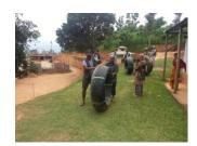
The project involves digging over a 1 km long trench, to lay the pipe to bring water from further down the hillside up to the school.
